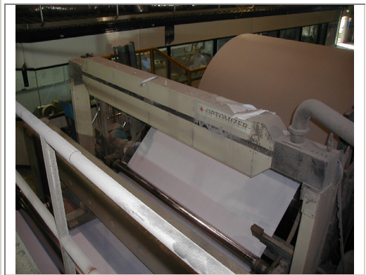
South East Asian Installation
