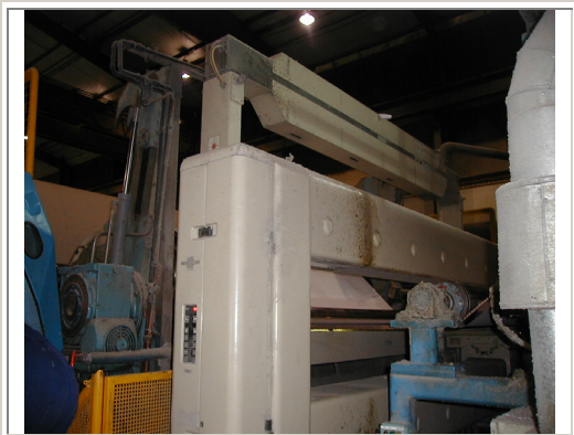
South East Asian Installation
